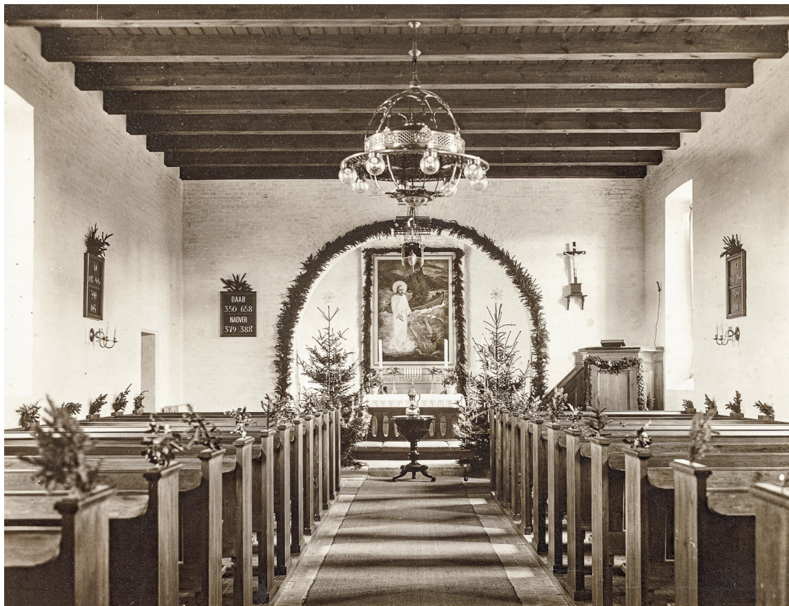
Fig. 10. Indre set mod nordøst, formentlig i 1960'erne. Foto Johs. Rasmussen. I Svanninge Folkemindesamling. – Interior looking northeast, presumably in the 1960s.
