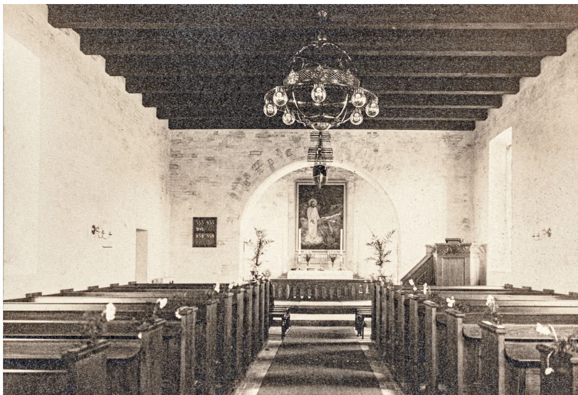
Fig. 19. Indre set mod nordøst, formentlig i 1930'erne. I Svanninge Folkemindesamling. – Interior looking northeast, presumably in the 1930s.
